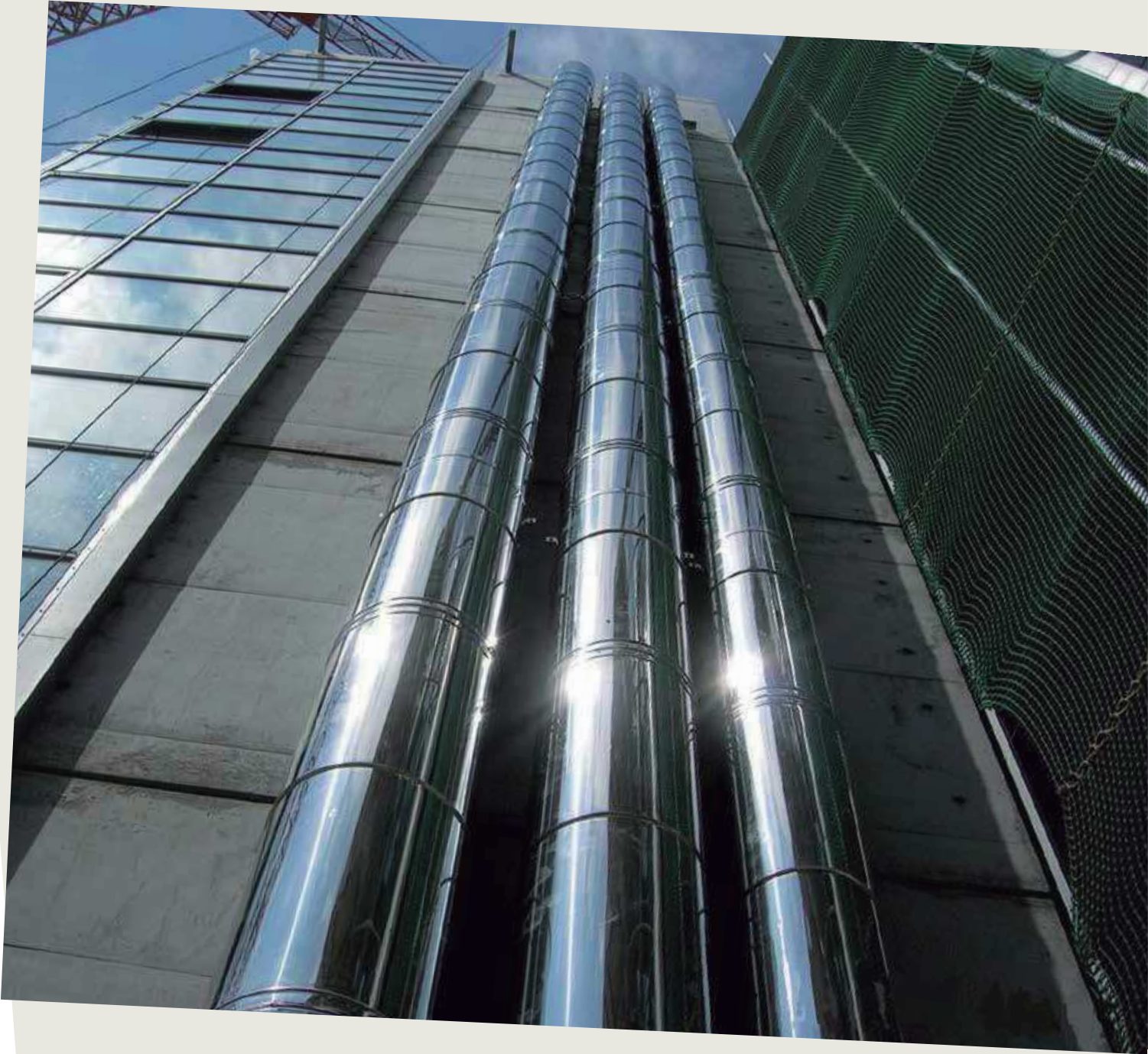
Conducto EI30 Gaine EI30 Duct EI30
